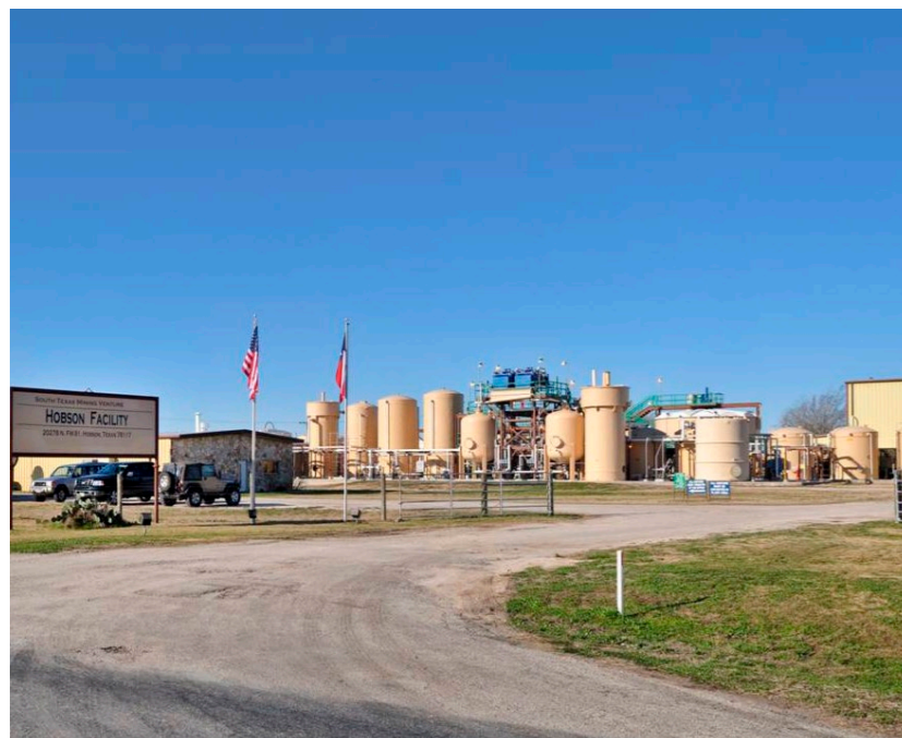
The Hobson production facility has been completely renovated and is state of the art. (Source: Uranium Energy)
